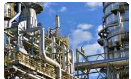
Kraftwerksbau | Power plant construction
